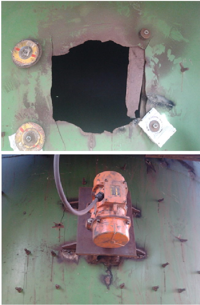
Fig. 1. Unsuccessful anti-gamming and damage of the silo wall due to non-efficient vibration.
